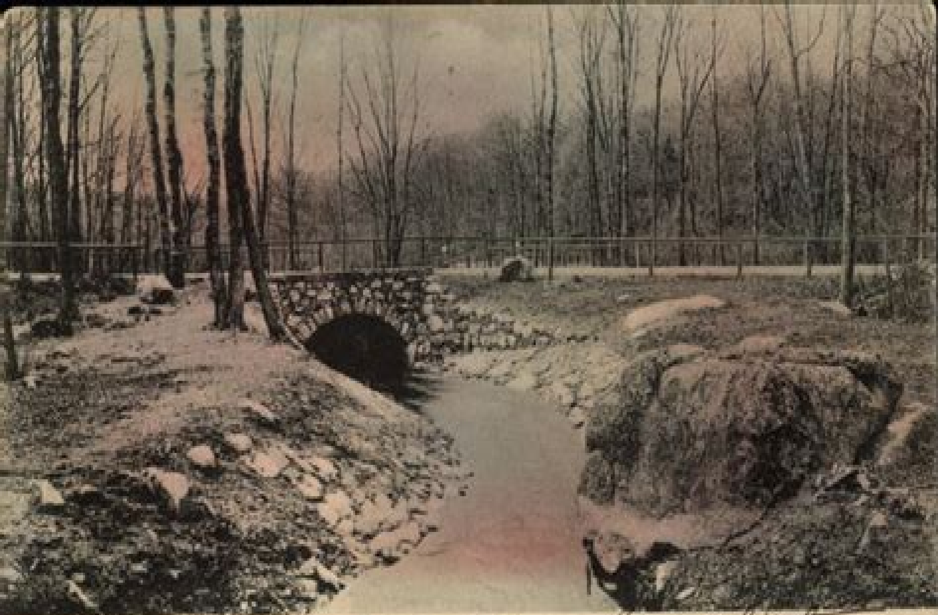
Bridge, Blue Hill Reservation, Milton, Mass.
